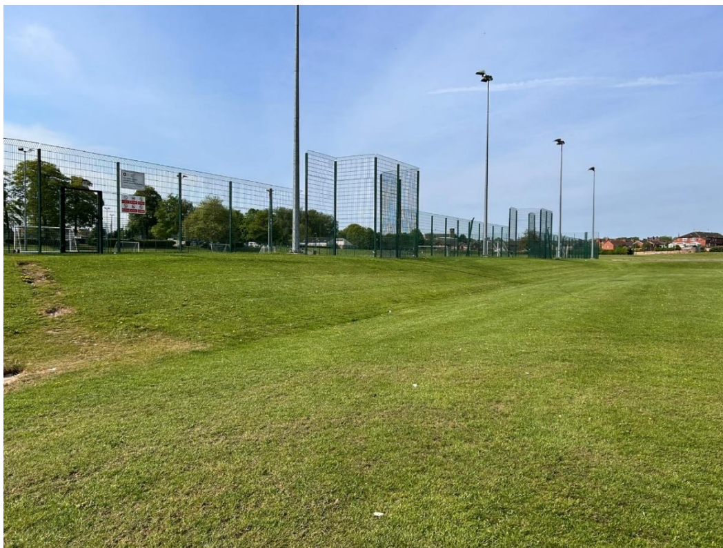
Photograph 1 - typical view of the amenity grassland surrounding the existing artificial pitch area (map reference 3).
